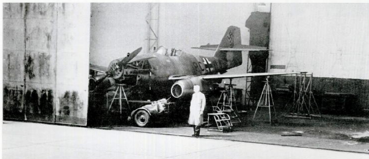
BELOW: During the early spring of 1942 the Me 262 V1 was fitted with a pair of BMW P.3302 V11-V14 engines, but these failed during the first attempted flight on 25 March. Wendel had to land the aircraft on the power of the Jumo 210 only. The BMW's were removed and the aircraft eventually re-engined with two Jumo 004 turbojets.
