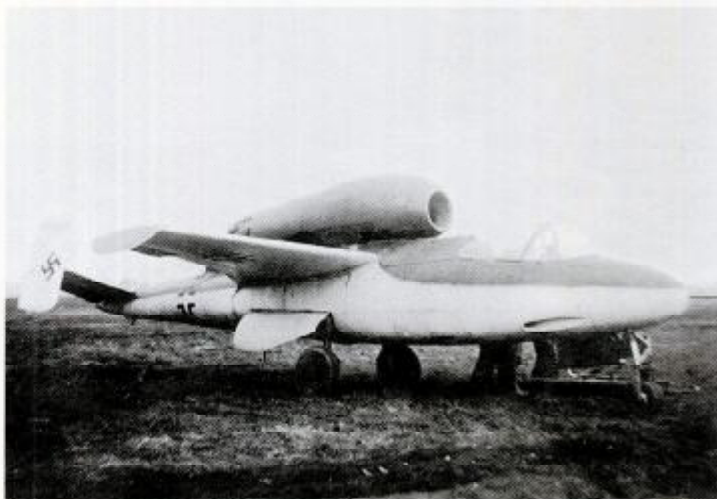
ABOVE: The Ju 248 V1 was completed in January 1945 and test flown as a glider from February. It was an extensively modified version of the Me 163 with a full vision canopy and a fully retractable undercarriage. The prototype failed to fly on the power of its twin combustion chamber rocket engine before the end of the war.
