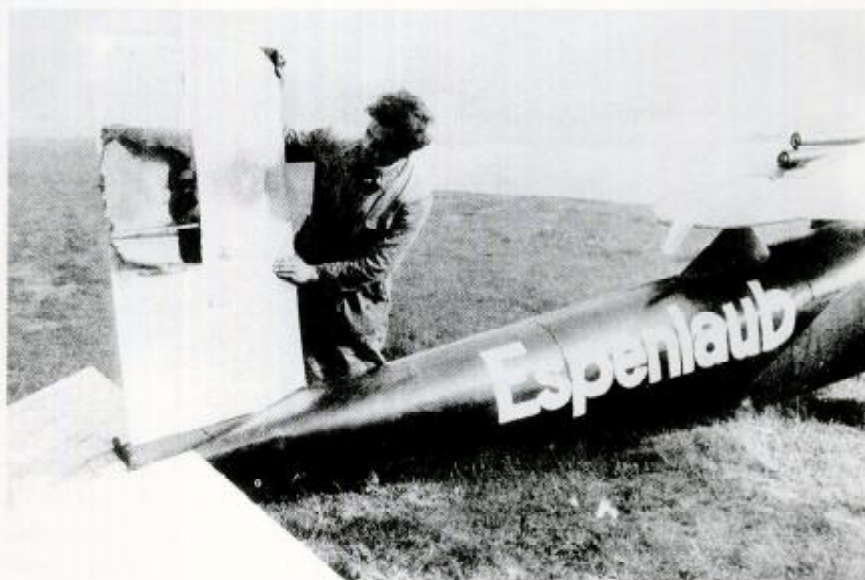
BELOW: Some of the hazards of early rocket flight! Gottlob Espenlaub examines the damage to the rudder of the E 7 which caught fire during a first test flight on 29 October 1929. Although he managed to land safely, the asbestos covering failed to prevent the damage shown.
