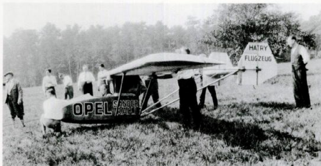
ABOVE: The tail-first Raab-Katzenstein Ente was the first piloted rocket-propelled aircraft to be flown in Germany. After several abortive attempts, the aircraft made its first 60-80 second flight on 11 June 1928 powered by two 20 kg (44 lb) thrust Sander engines. A second flight on that day was abandoned after one of the engines exploded, and set light to the rear fuselage.
